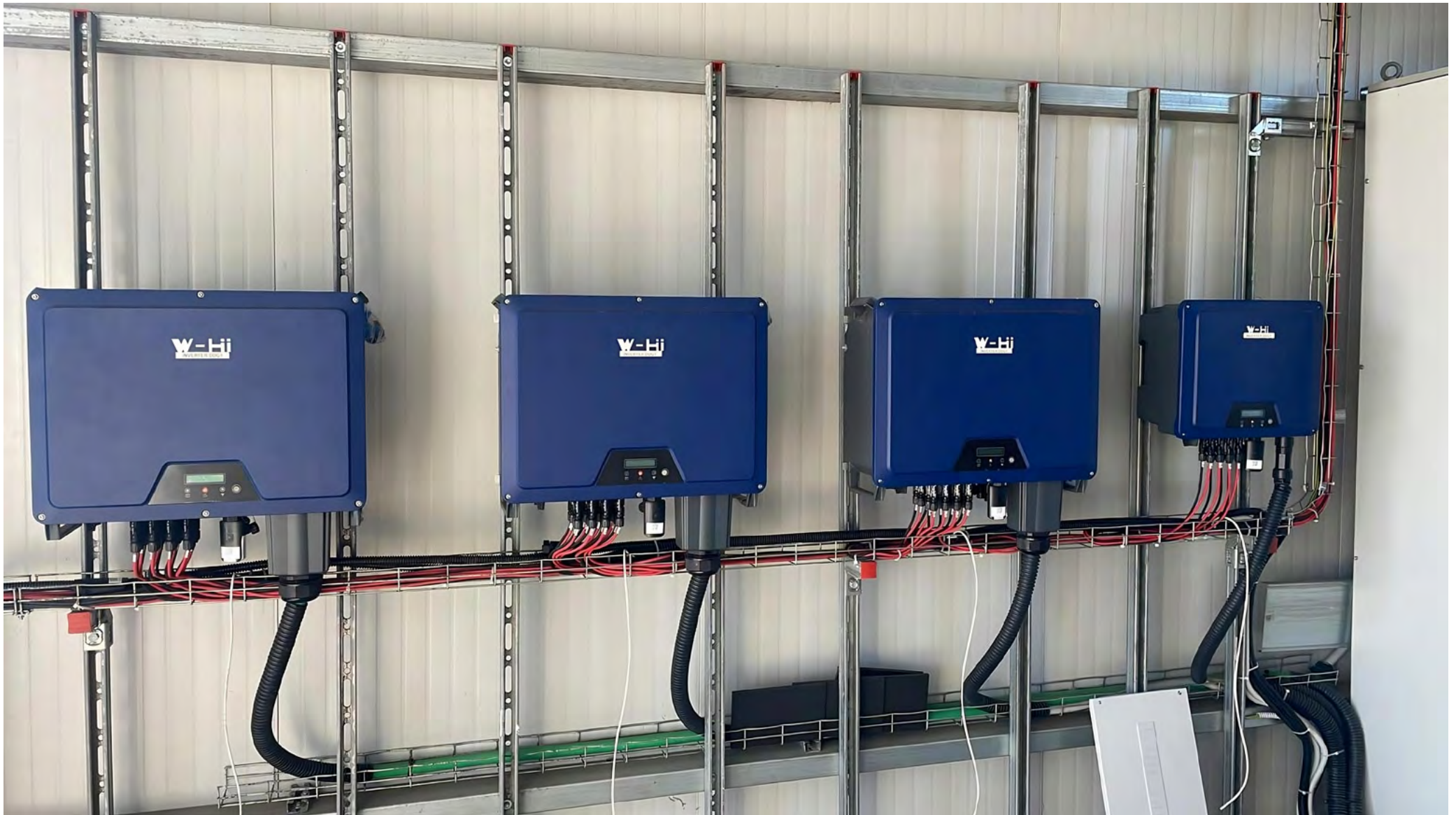
INVERTER W-Hi W-HPT 50-30-20 kW with management via W-Hi Manager Datalogger. Sassari - Italy
