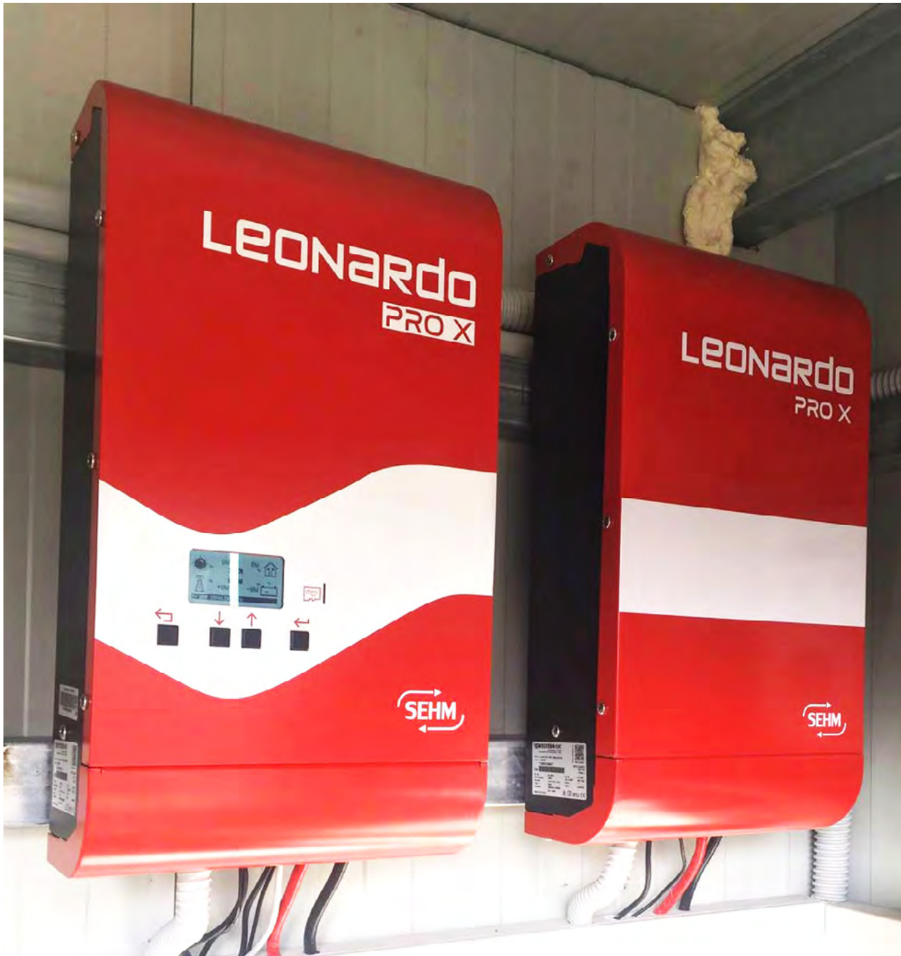
Leonardo Pro X Master + Slave with WRM9 - Smart Slave MPPT 90A 12/24/48V charge controller Italy
